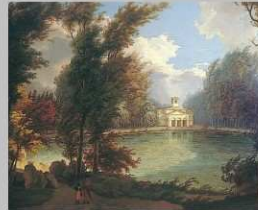
The Engine House and pond (1809)
